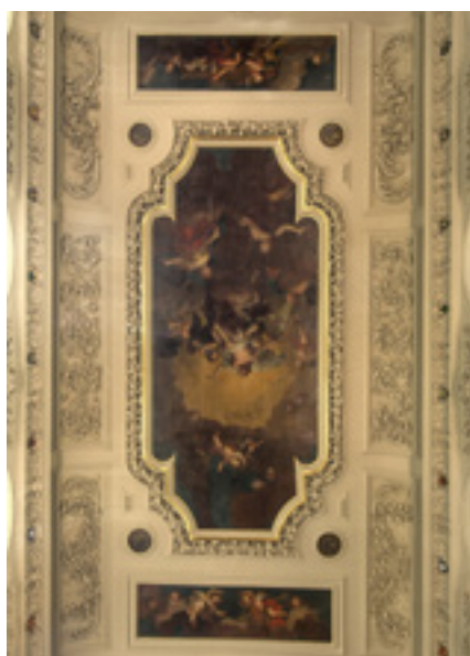
Detail of the ceiling paintings and plasterwork after cleaning and revarnishing
