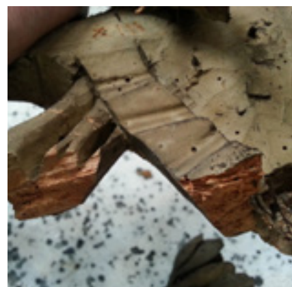
Woodworm damage in carvings of the reredos
