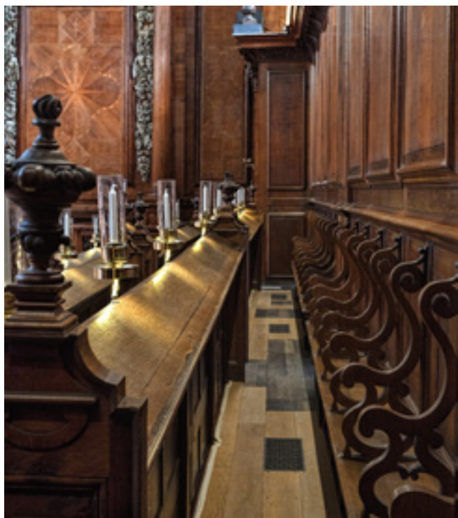
Repairs to the raised floor below the pews, with a mixture of new European oak boards and sections of salvaged originals
